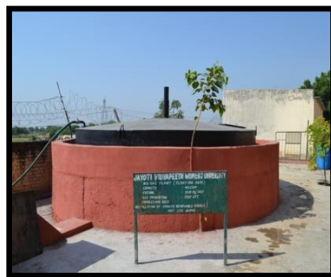
Bio Gas Plant
