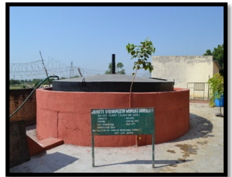
Bio Gas Plant
