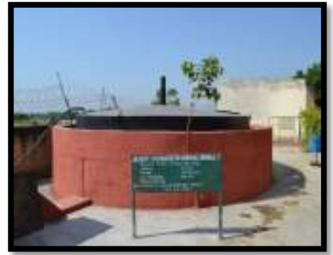
Bio Gas Plant
