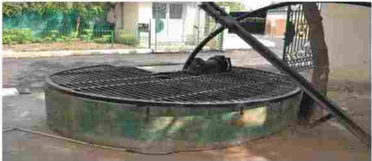
Open Well for Collection of Rainwater
