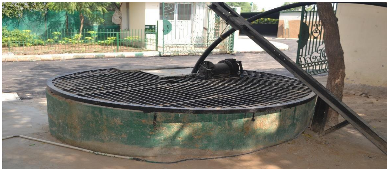
Open Well for Collection of Rainwater
